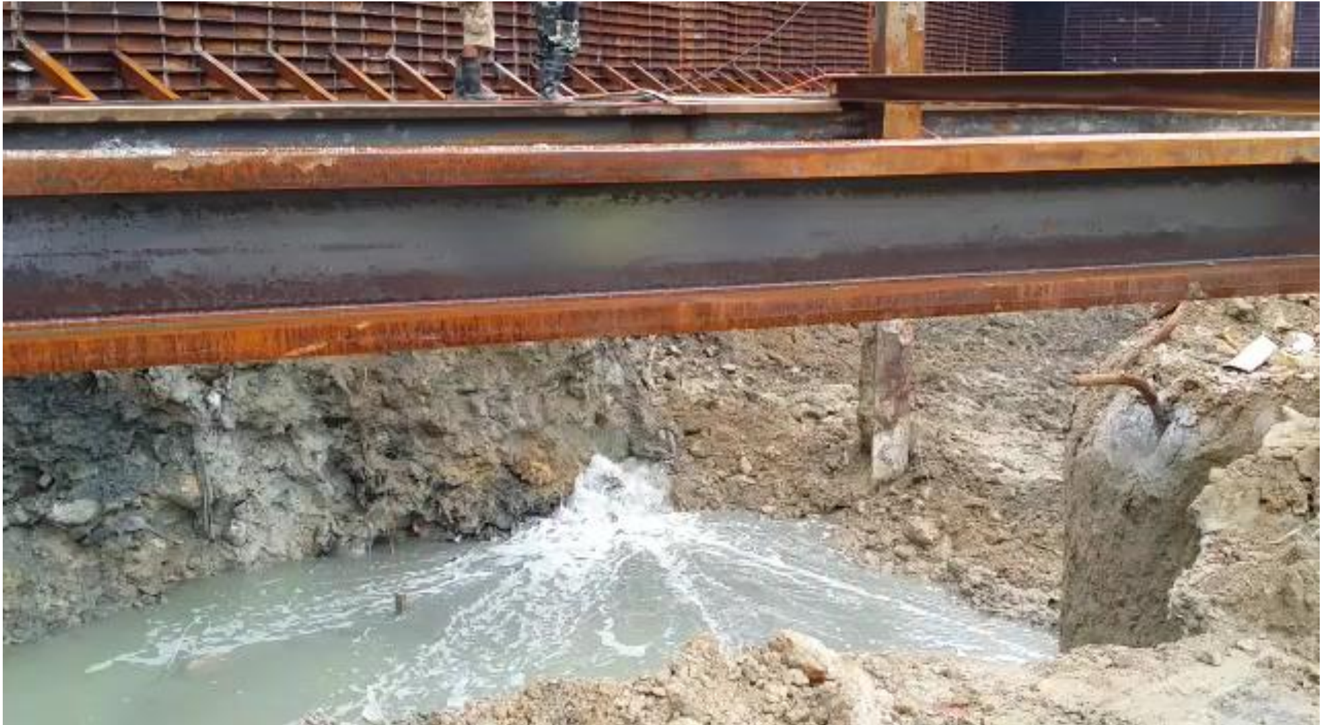
TAM Grout Treatment Zone
